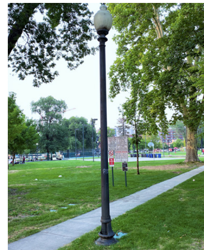
S1. Small light pole
