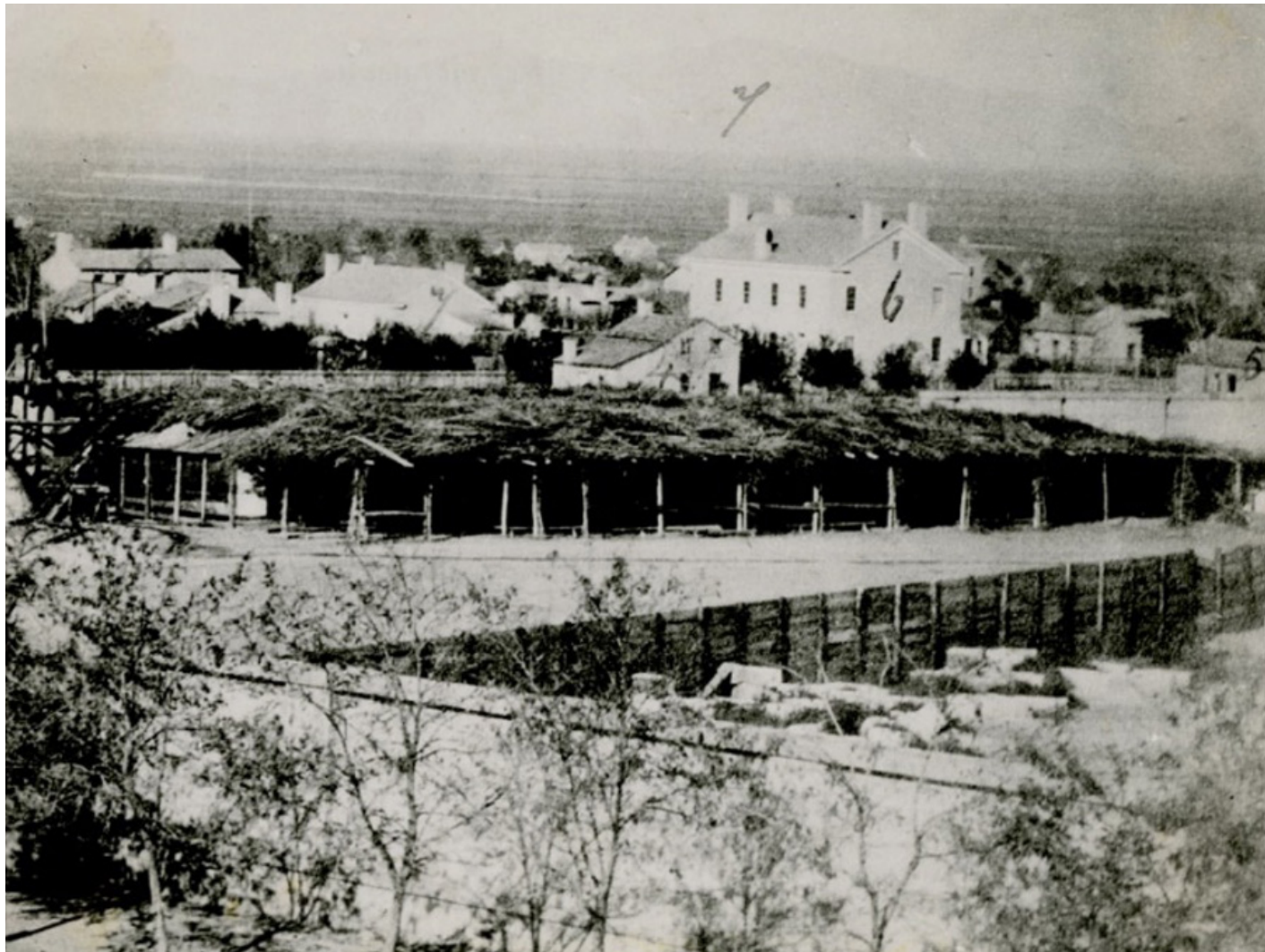
Figure 2-11. A later bowery built on the temple block shows the general style of what the fort bowery may have looked like. (R-3-Z)
