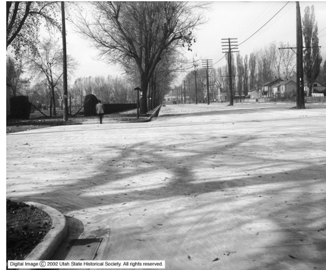
Figure 4-1. 1909 photo of street paving looking west along 300 South. Pioneer Park is visible on the left-hand side of the historic image. This photo illustrates the sidewalk, park strip and street tree configuration defining the perimeter of the park. A clipped hedge lined the inside of the public sidewalks. The corner entrance to the park is visible.
