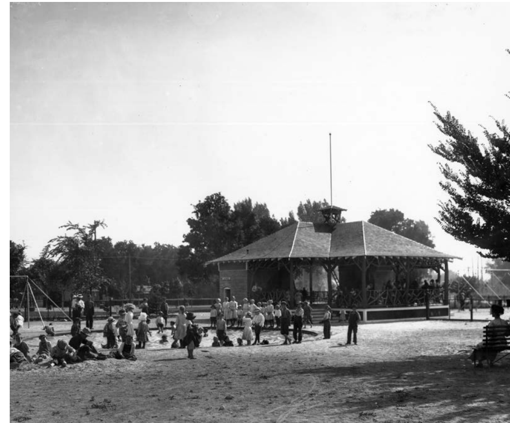
Figure 4-9. 1911 photo looking southwest with the pavilion in the center-right of the image, wading pool center-left of image and playgrounds visible in the background on either side. A short, visually open fence is visible in the background defining the playground spaces and can be seen extending north from the center of the pavilion. A park bench is visible on the right-hand side of the image. While the foreground appears to be dirt or sand, the background contains mown lawn, and large open-branching shade trees, in a scattered picturesque configuration.
