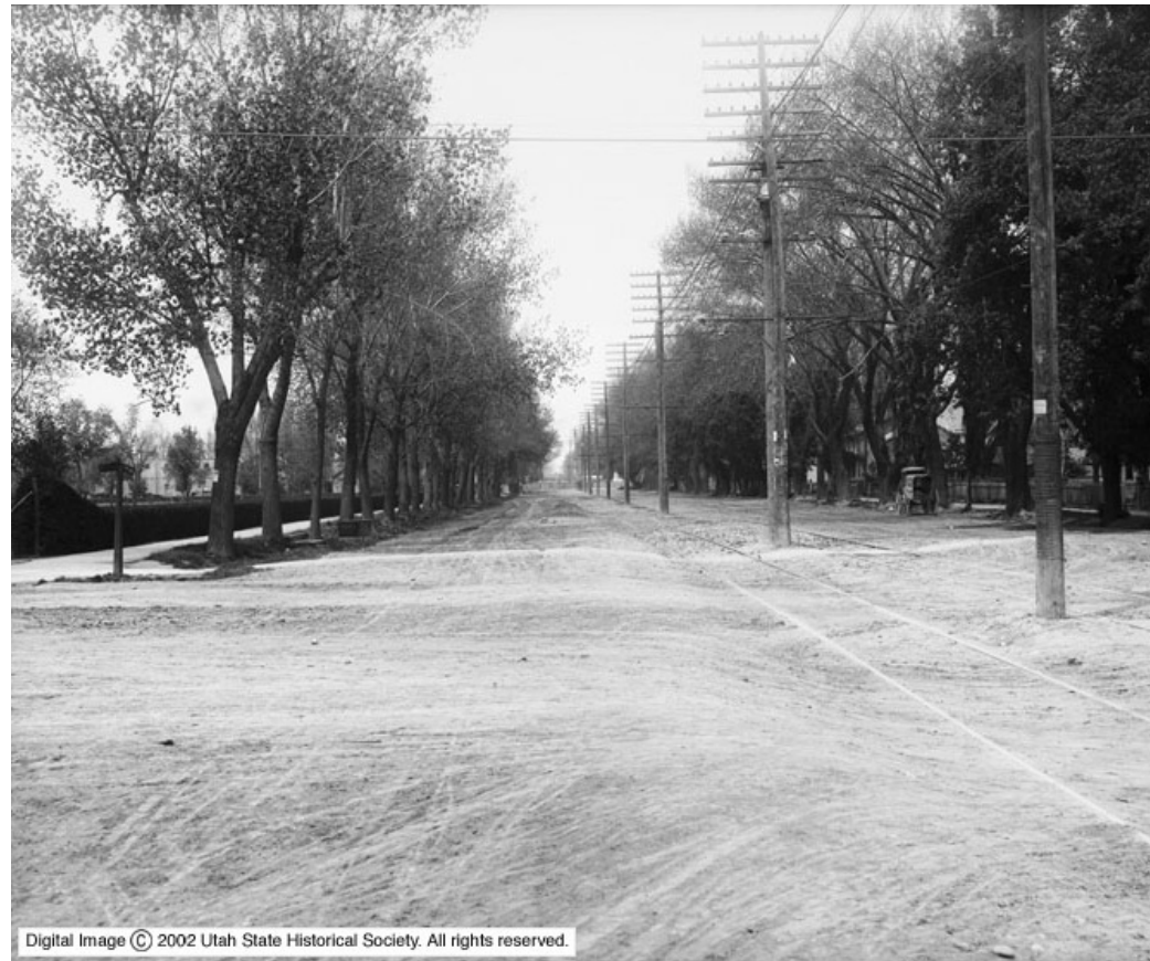
Figure 4-3. 1909 photo of street paving looking south along 400 West. Pioneer Park is visible on the left-hand side of the historic image. This photo illustrates the sidewalk, park strip and street tree configuration defining the perimeter of the park. A clipped hedge lined the inside of the public sidewalks. A portion of the corner entrance to the park is visible.
