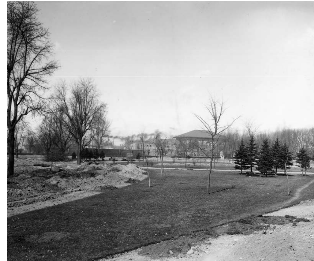
Figure 4-5. Late 1910 photo looking northwest across the park, with the Denver & Rio Grande Depot visible in the background. The piles of dirt visible in the foreground and on the left indicate that this image was taken mid-construction.
